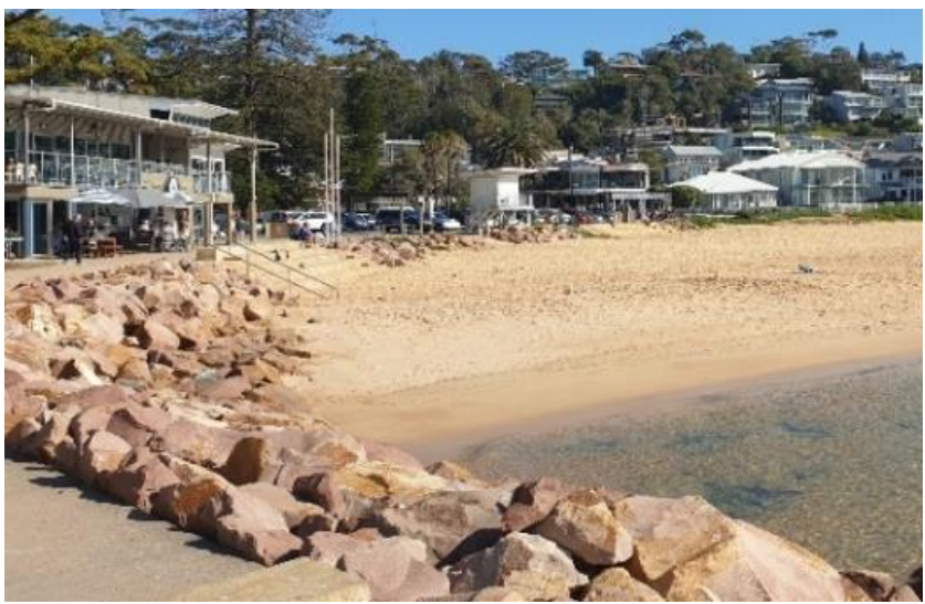
Examples of coastal protection structures. Left – Terrigal Seawall, right – Avoca rock revetment
