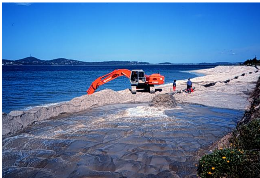
Sand Nourishment. Left: Jimmys Beach NSW. Right: “Rainbowing” – dredge pumping nourishment sand from offshore into the active beach zone (NSW Reconstruction Authority State Disaster Mitigation Plan, 2023)
