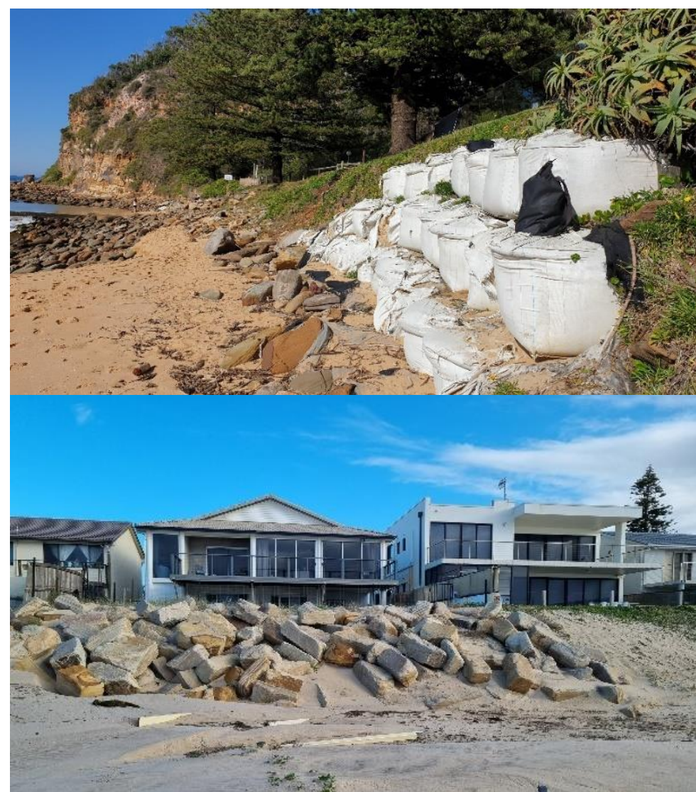
Ad-hoc coastal protection works – Top MacMasters Beach SLSC; bottom – Curtis Parade, The Entrance North
