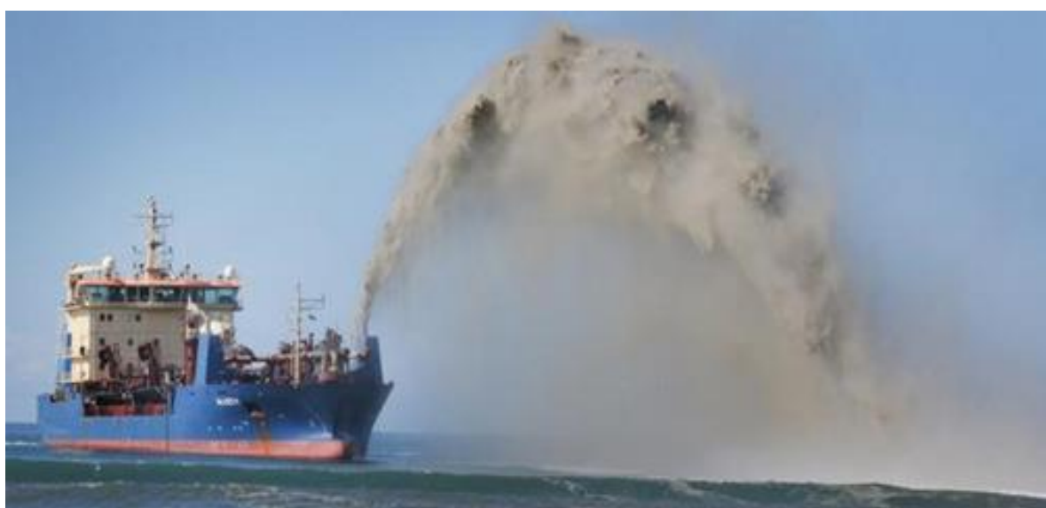
Sand Nourishment. Left: Jimmys Beach NSW. Right: “Rainbowing” – dredge pumping nourishment sand from offshore into the active beach zone (NSW Reconstruction Authority State Disaster Mitigation Plan, 2023)
